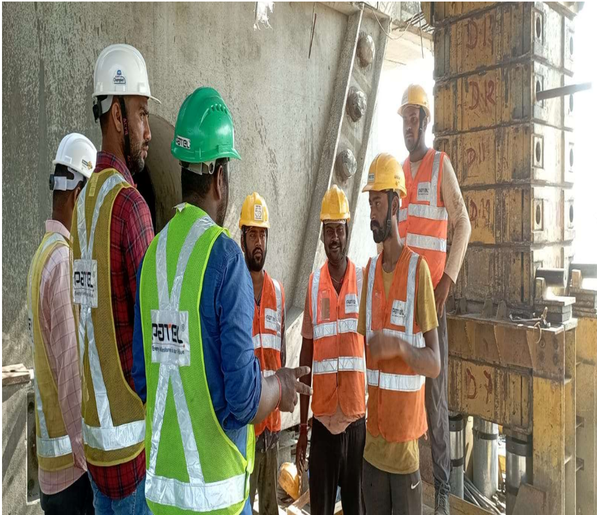
Safety instructions given to labours at Km.107+400 (Major bridge)
